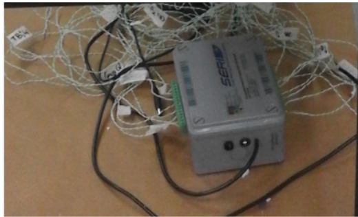
Figure 6. Data Logger ADAM-4019 for temperature data
