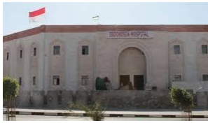
Figure 8: Indonesia Hospital at Gaza Strip
